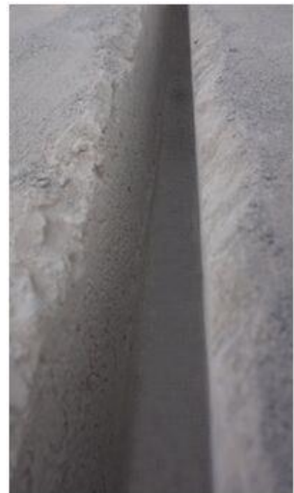
On-site cutting trench
